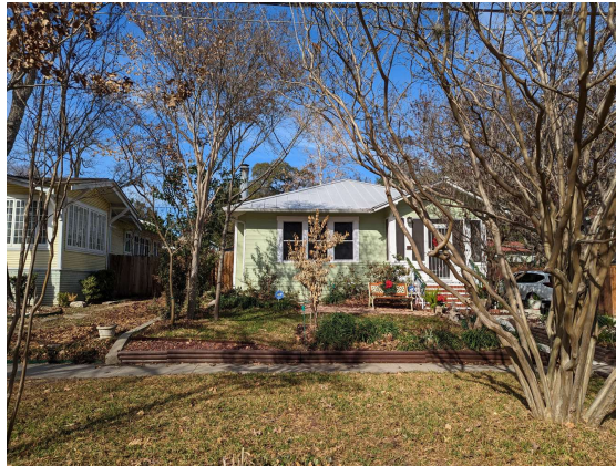
Ⓒ 111 W. HUISACHE HIPPED METAL ROOF WITH RIDGE CAP
